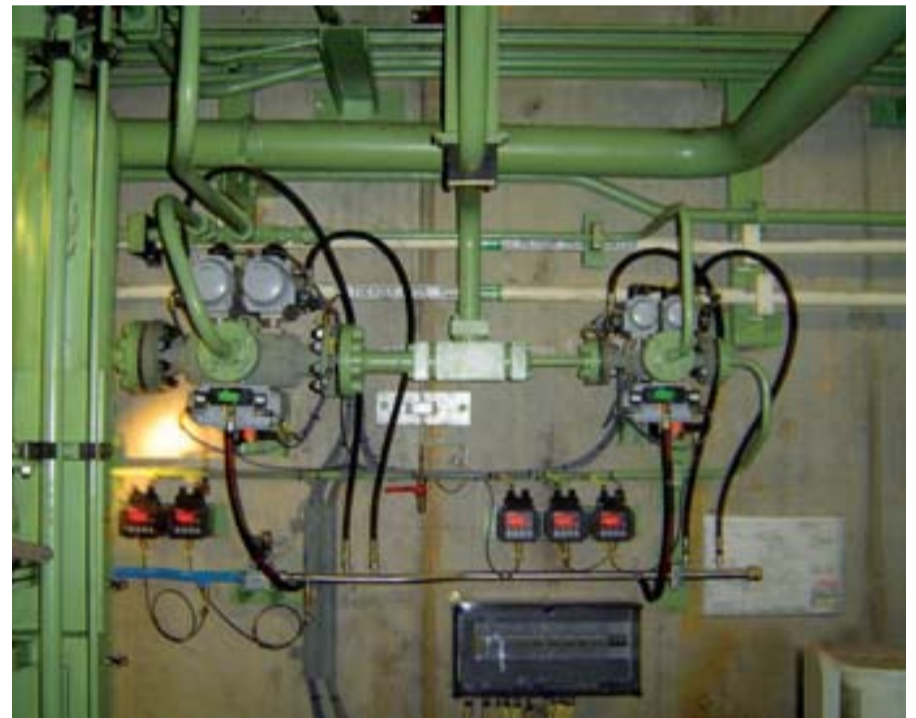
Trunnion mounted multiport twin ball valves supplied as safety valve on high pressure hydraulic system.
